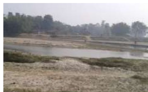
Fig. 9 cross drainage work site across River Kankai
