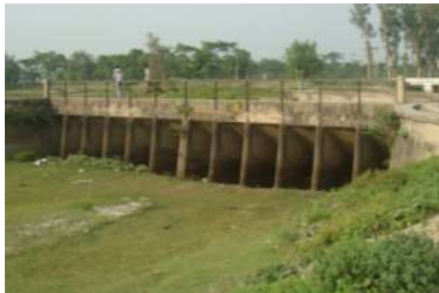
Fig. 3 Syphon Acqueduct at Sitadhar.
