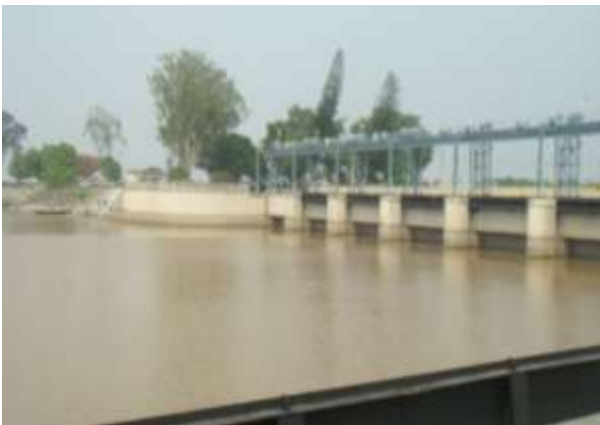
Fig. 2 Head Works of Eastern Kosi Canal.
